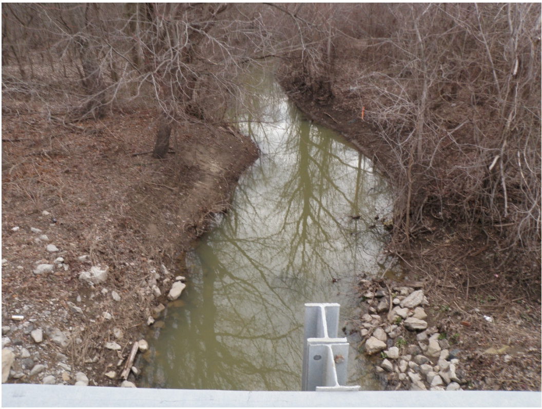
STR-1 Looking Upstream
